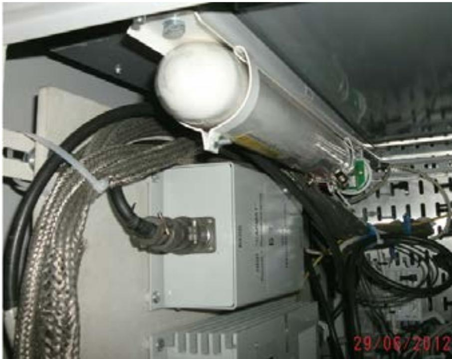
Photo 4 – Self-activated powder extinguisher OSP-1 and the “Fire detector” (IP101-V, located to the right of OSP-1) in the device compartment cab, cover is opened (photo V.O.Bulatov).
