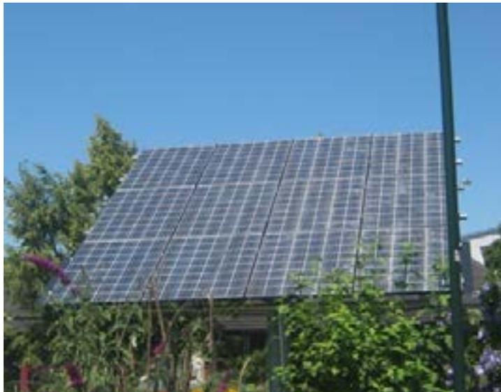
*Figure 4. Amorphous silicon photovoltaic panels*
