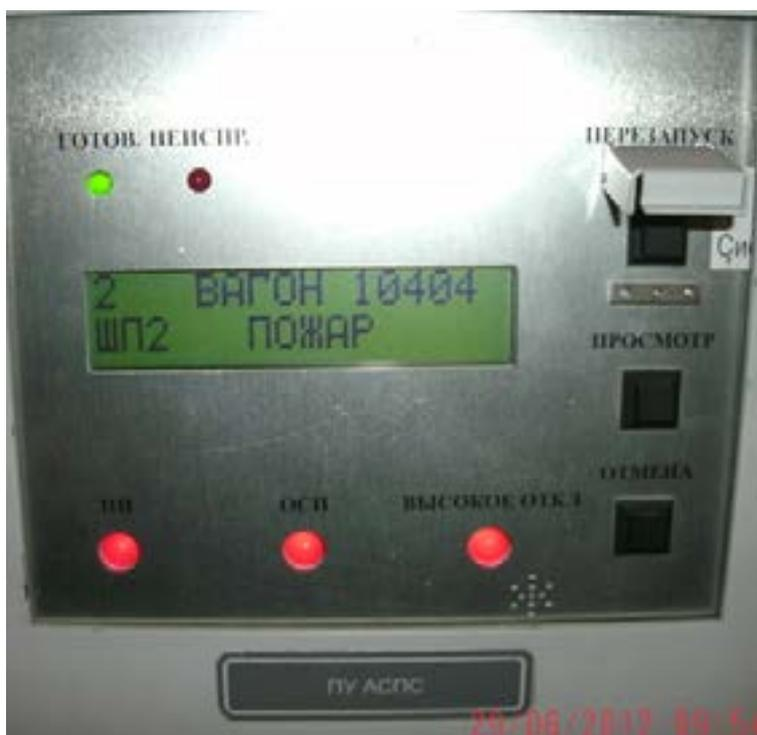
b) Information on the remote ASPS when testing the system fire alarm
